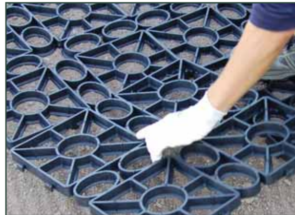
Simple and fast laying of the GEOFLOR grid.
