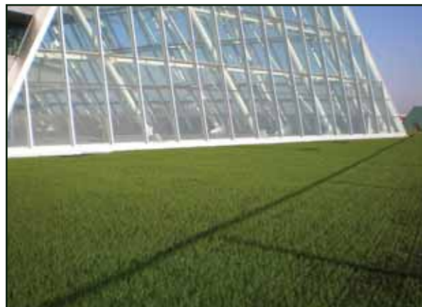
20 days after the installation of GEOFLOR : grass partially incorporates the grids.
