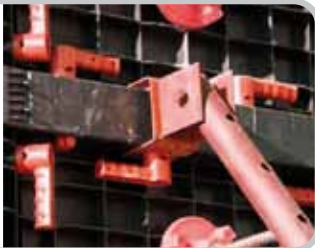
Formwork stabilizer joint
