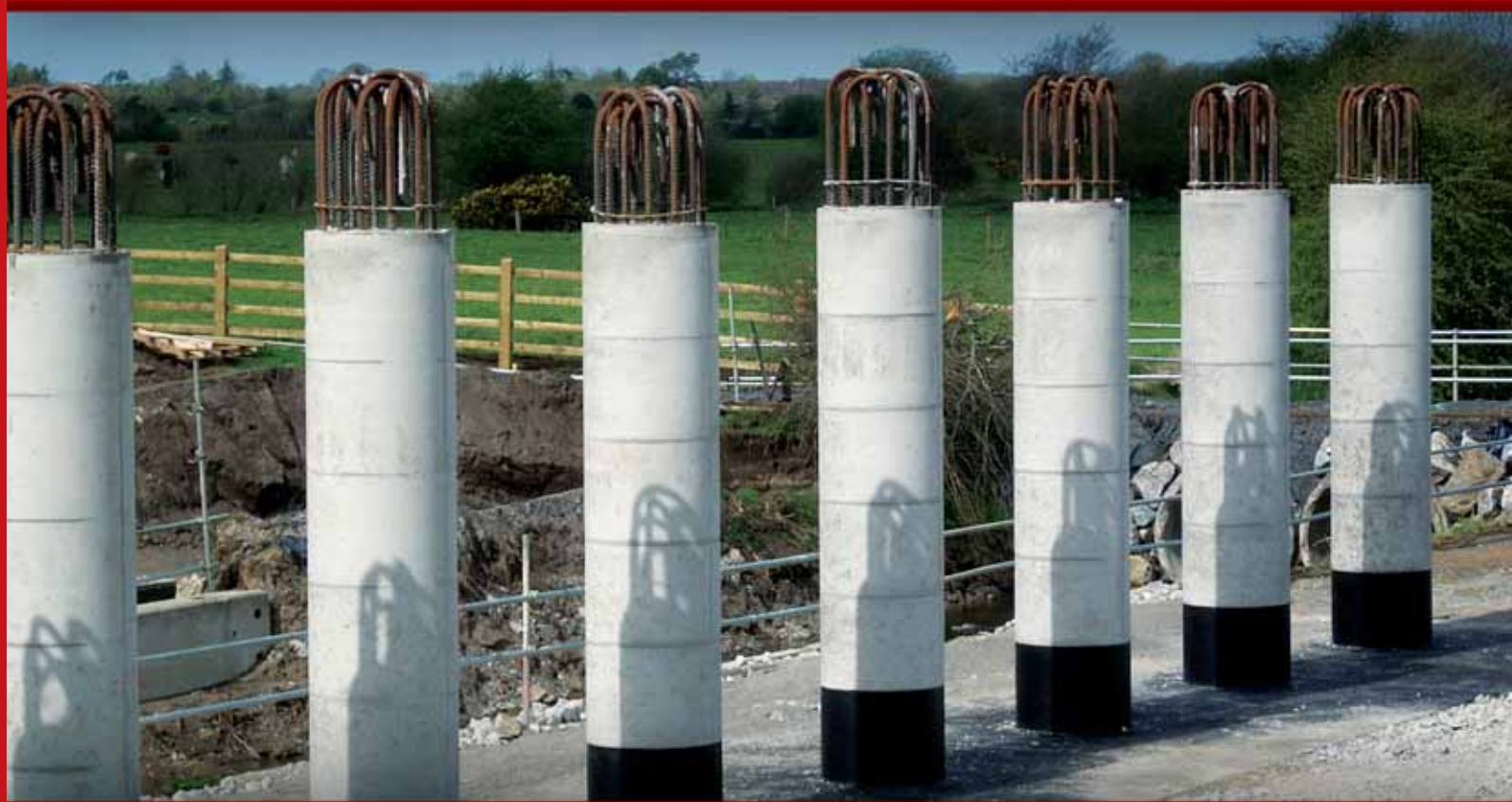
The 1 st plastic formwork for round columns
