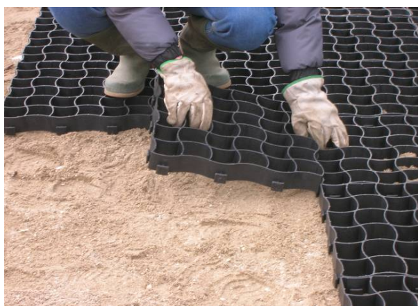
Fig. 1 Grid locking
