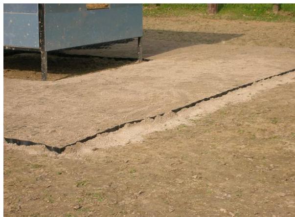
Fig. 3 Sand filling
