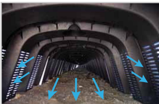
figure 2) Bottom and side drainage.
